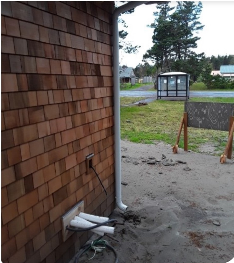
Gutters are up and working.
