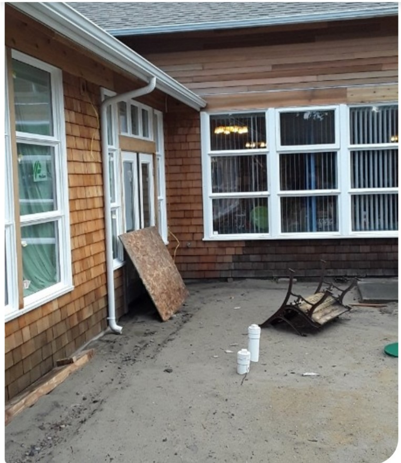
Siding on old and new building finished Waiting for stain
