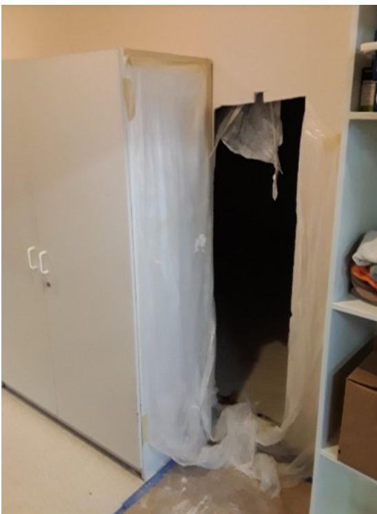
Waiting for new doors for storage room.
